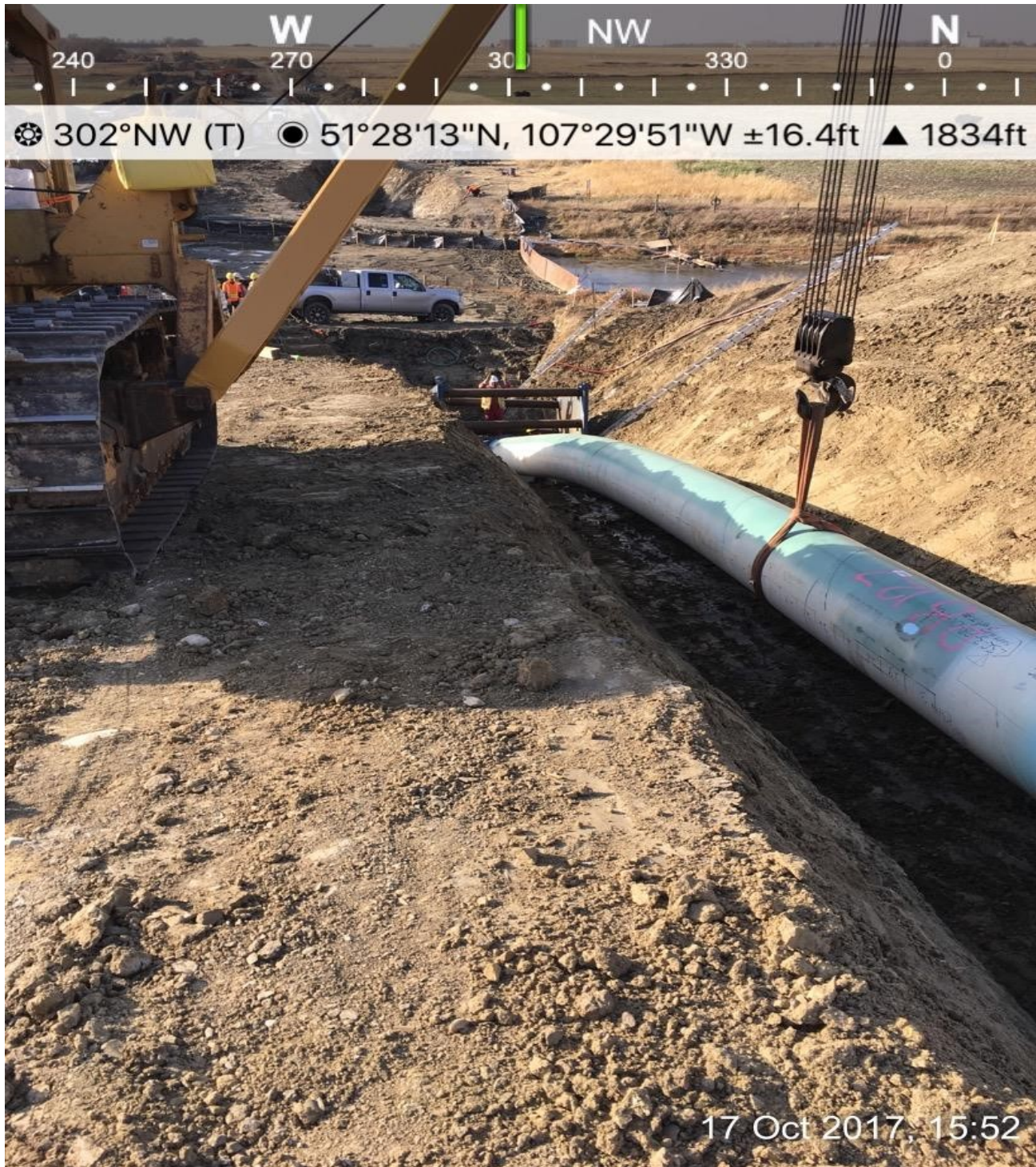
Tie in pipe at McDonald Creek
