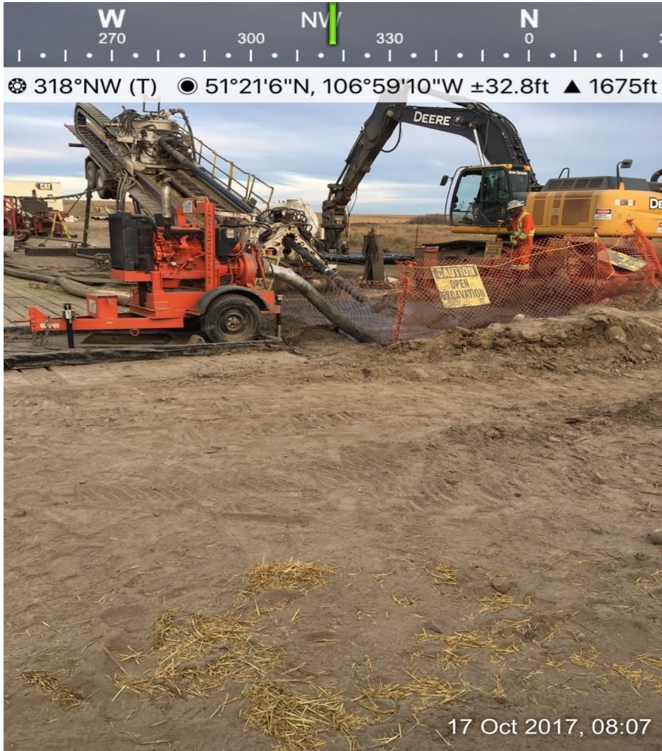
Horizontal directional drilling rig at South Saskatchewan River
